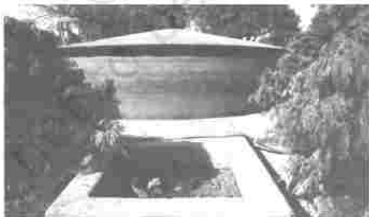
Fig. 7.4 Gobar Gas Plant uses cattle dung to produce energy
